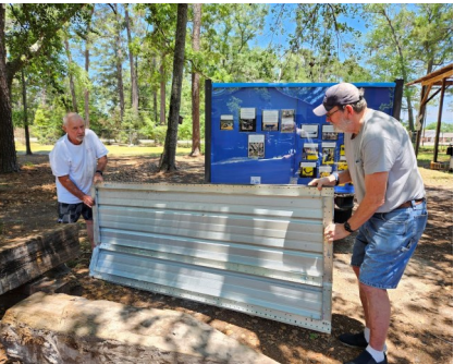
Installing outside exhibits
